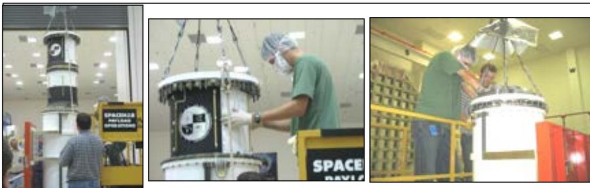
Figure 15-4: PSC engineers perform a vertical integration (CAPE-ICU-I)
