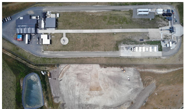
CONSTRUCTION OF ROCKET LAB'S LC-1 PAD B | January, 2020
