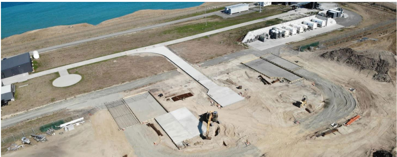
CONSTRUCTION OF ROCKET LAB'S LC-1 PAD B | March, 2020
